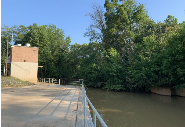
Raw Water Intake at Jacob's Fork
