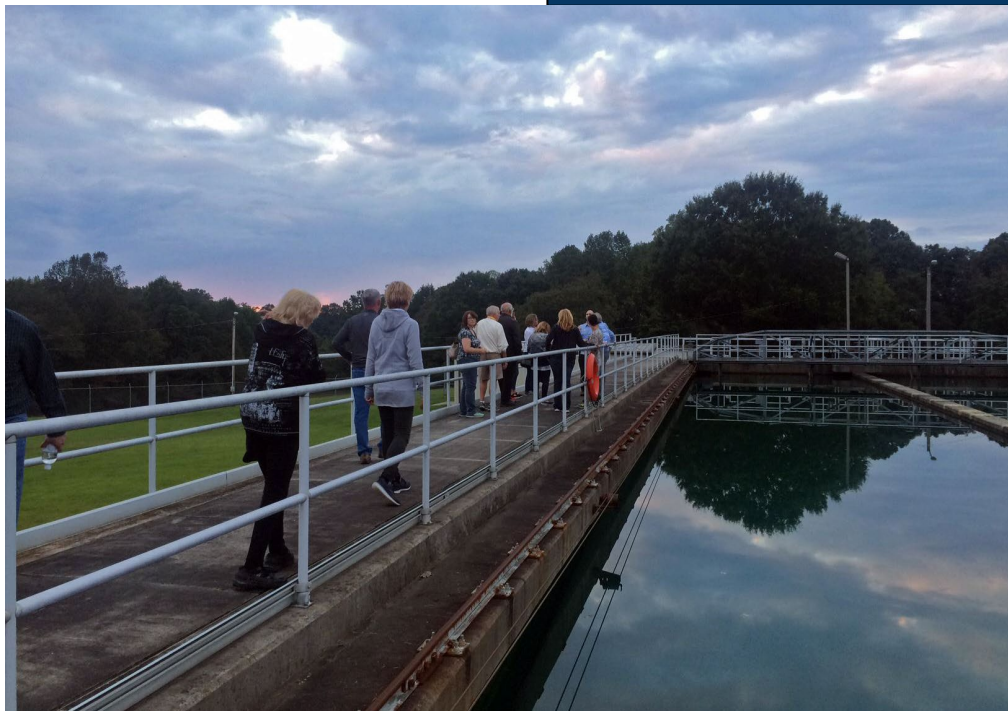
Newton’s Water Treatment Plant
